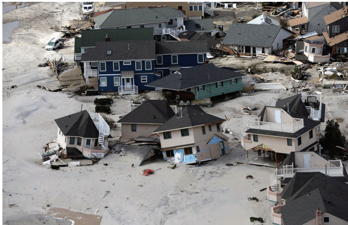
FIGURE 1.2 Hurricane Sandy A portion of the New Jersey shoreline shortly after this huge storm struck in late October 2012. The storm was especially destructive because it struck a region with a high population density and extensive development. Shifting shoreline sands and the desire of people to occupy these areas are often in conflict. (Photo by AP Photo/Mike Groll)
